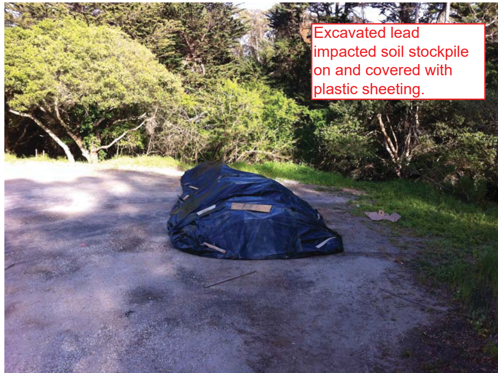
Dust suppression during excavated lead impacted soil stockpiling on plastic sheeting.
