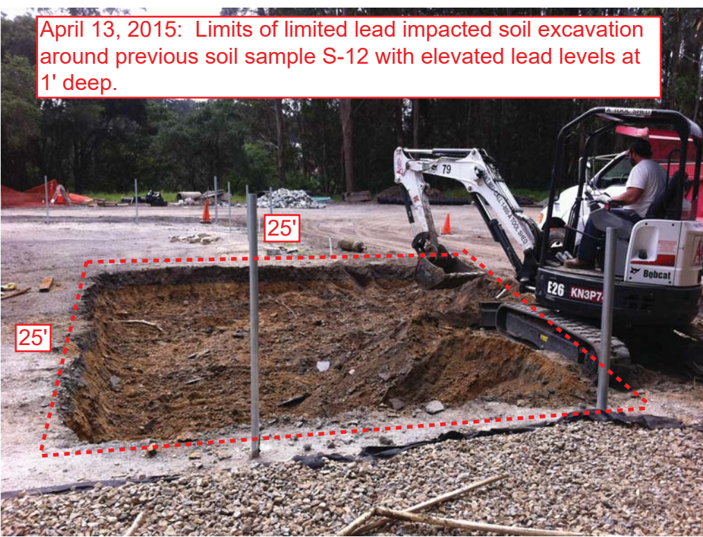
Sidewall sample depth targeting the coarser material based on original 1' deep samples.
