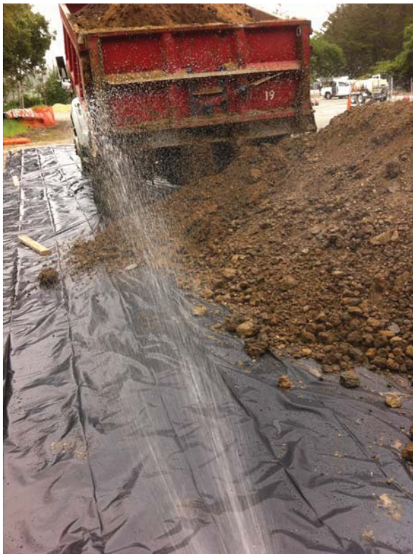
Dust suppression during excavated lead impacted soil stockpiling on plastic sheeting.
