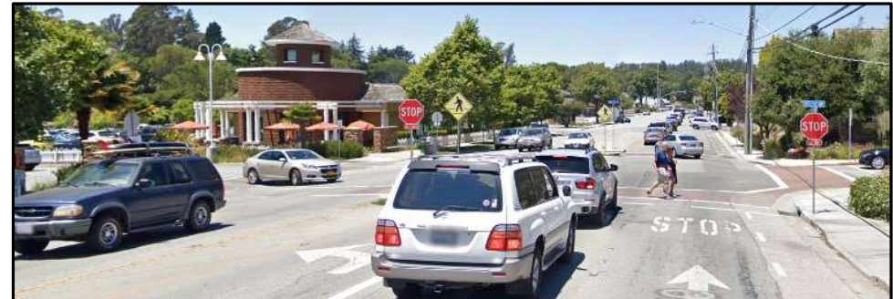
Multiple turn conflicts, long ped crossing distances
