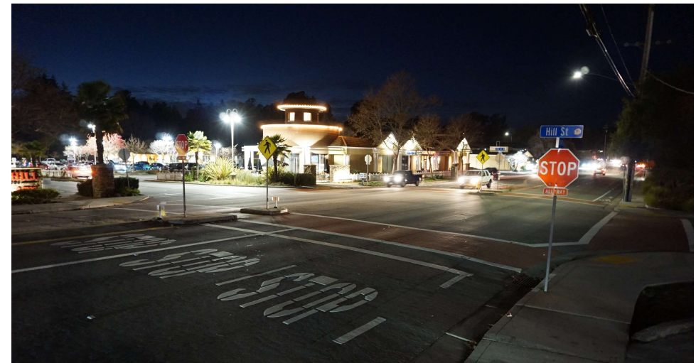
Limited crossing visibility and lighting
