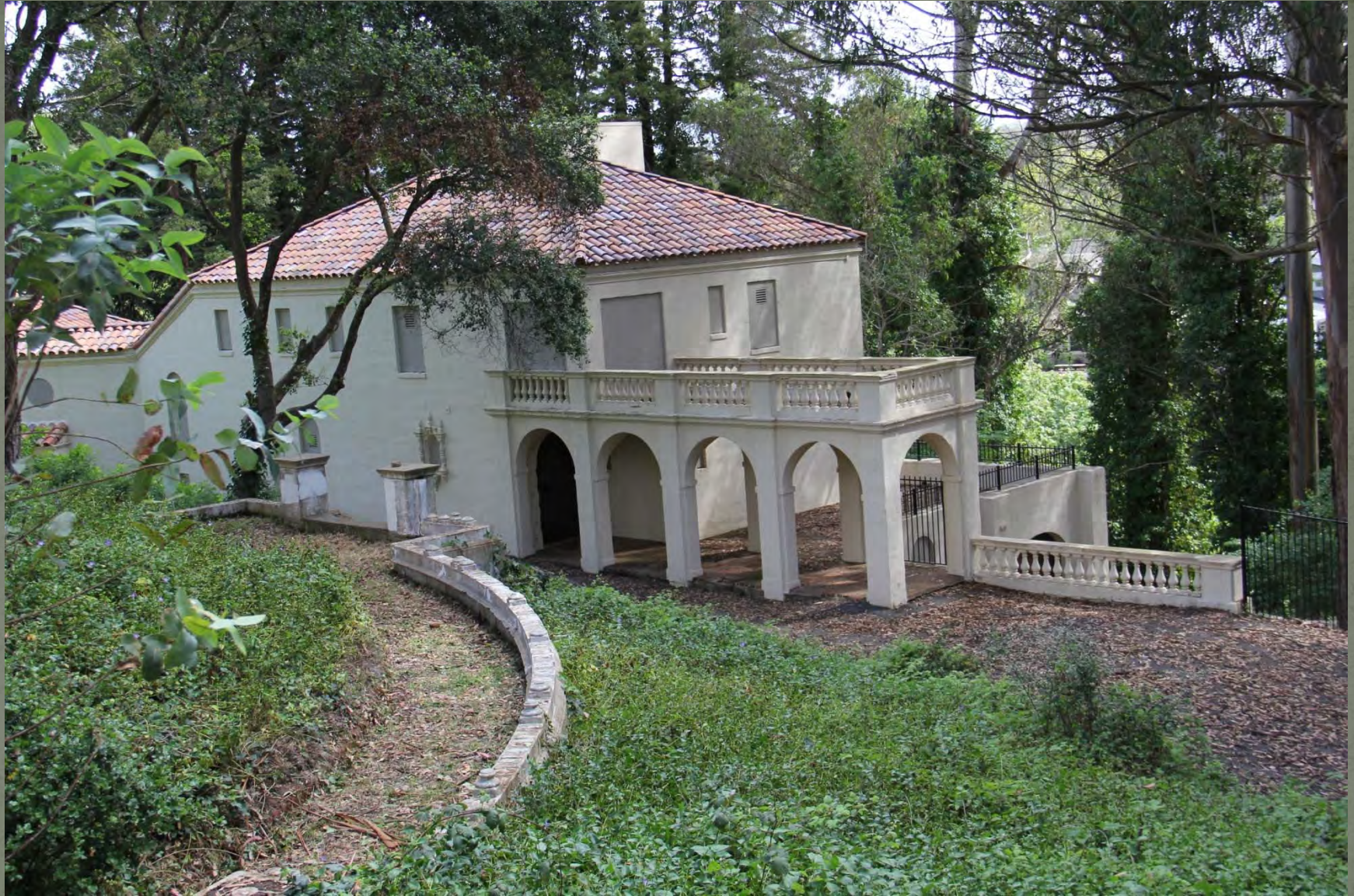
Location of balustrade rail overlooking mansion to be reconstructed
