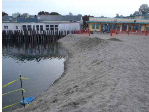
16-Inlet, Looking East
