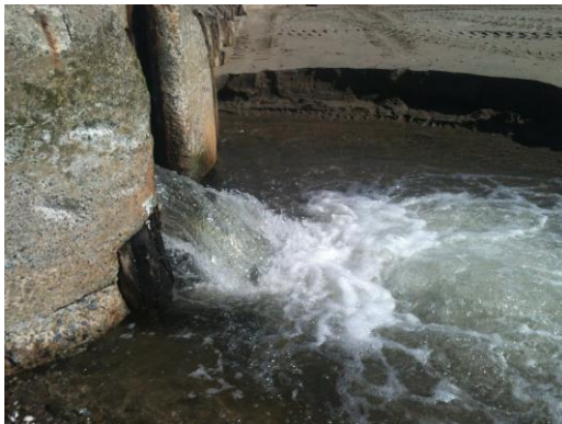
17- East Side Outlet Open
