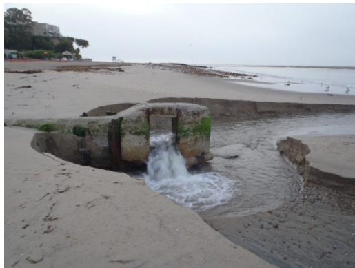
14-Outlet, Looking East
