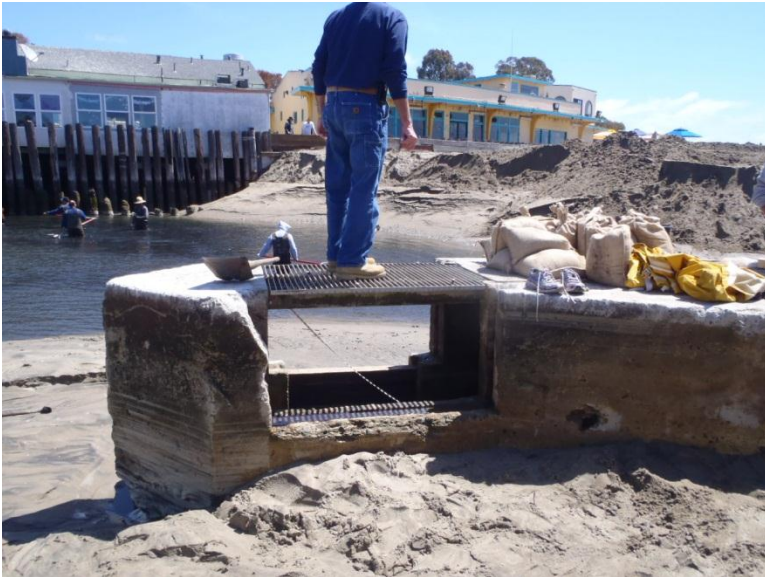
1)-Inlet at sta 225
