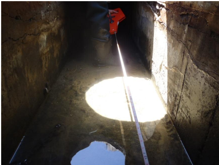
11) Sta 128 Floor and Sides
