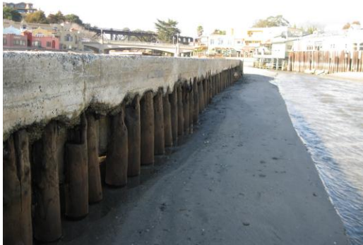
5- East Side Flume, Looking North
