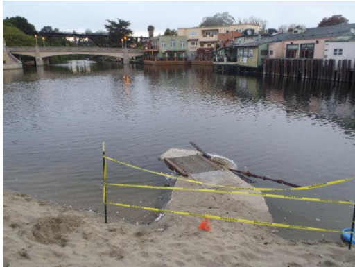
15-Inlet, Looking North
