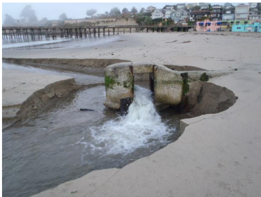
13-Outlet, Looking West
