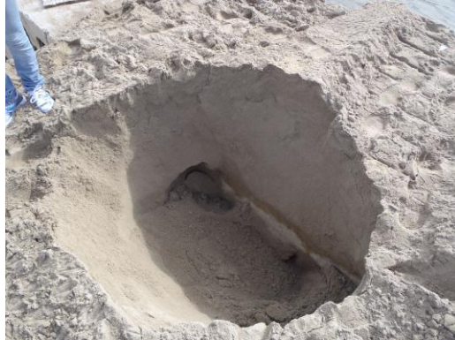
10-Sink Hole Near Inlet
