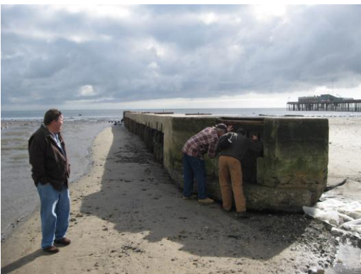
3-East side of Flume, Soquel Creek Open
