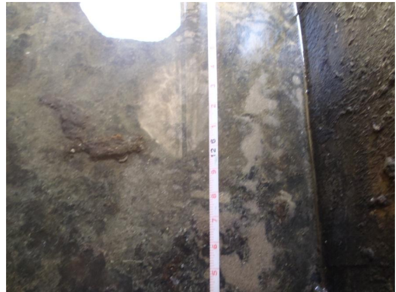
12) Sta 128 Floor, No Visible Cracks
