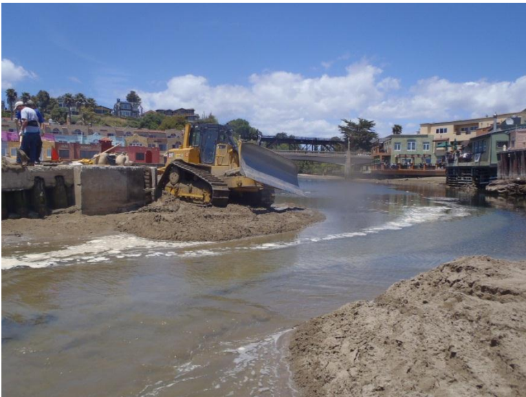
27) Lagoon Breach Prior to Closure
