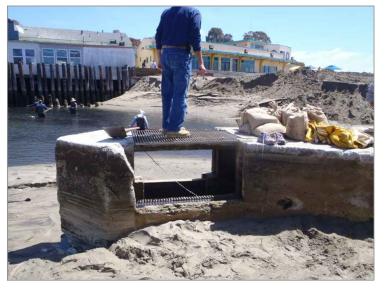
INLET AT STA 0+00
