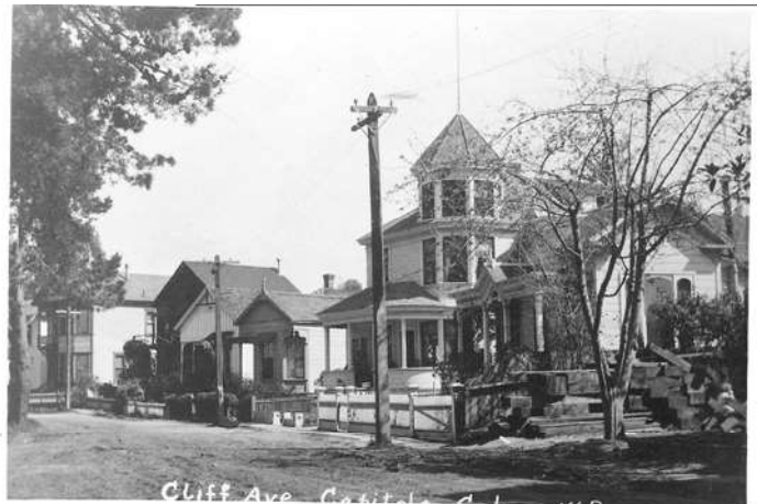
San Jose architect Jacob Lenzen designed his summer home on Cliff Avenue with a view tower. The Queen Anne style house was later owned by baseball star Harry Hooper. (Courtesy of the Lynn and French families)
