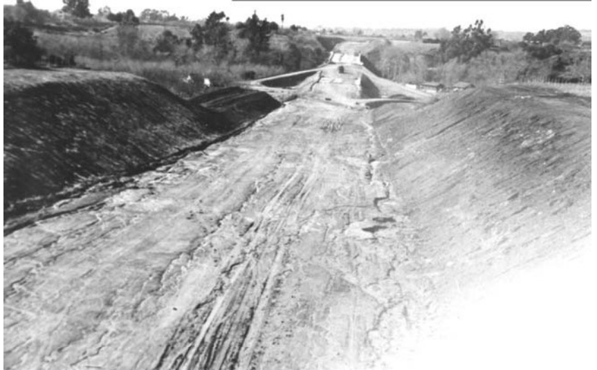
Highway 1 under construction, 1948 ( Courtesy of the Daubenbiss family )
