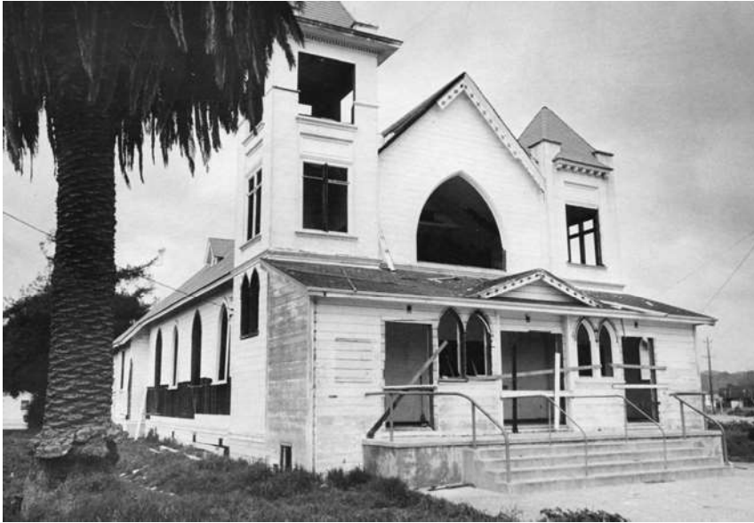
St. Joseph's Catholic Church, located at Bay and Capitola Avenues, was demolished in March 1973. (Capitola Museum)
