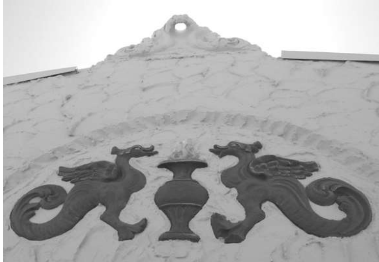
Venetian Court architectural detail
