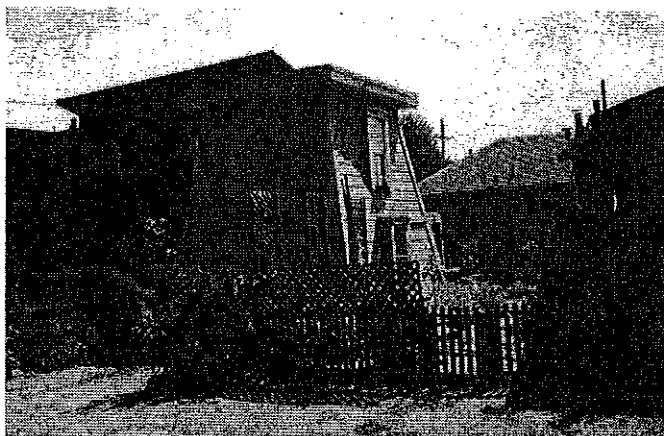
Emerald Street at 49th Avenue Utilitarian c. 1895
