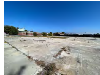
C EXISTING SITE CONDITIONS EXISTING BUILDING DEMOLISHED, FOUNDATION REMAIN
