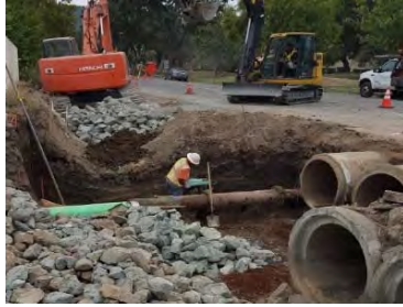
Yountville Hopper Creek Improvement Project
