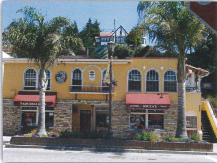
street lighting, planting, hardscape Michael Arnone + Associates, Capitola Village
