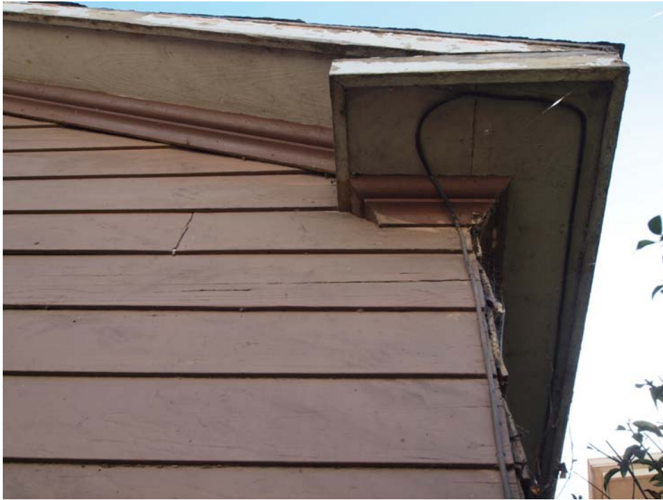
Detailed view of eave, viewed facing southwest.
