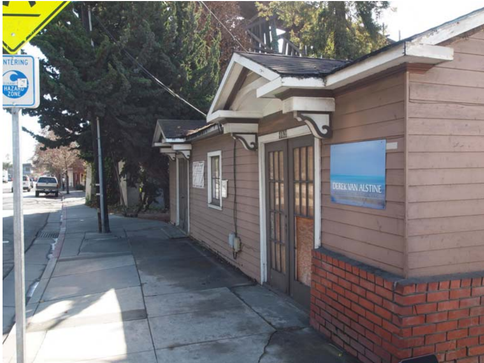
Street façade along Capitola Avenue, viewed facing southeast.
