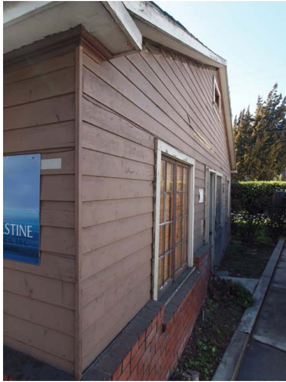
Right side elevation, viewed facing southwest.
