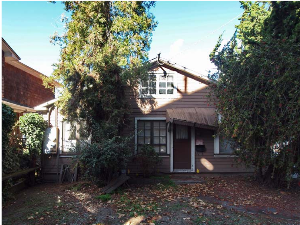
Left side elevation, viewed facing northwest.
