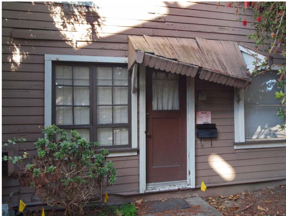
Detailed view of left side entry, viewed facing northwest.
