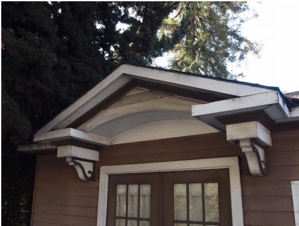
Detailed view of door hood, viewed facing south.
