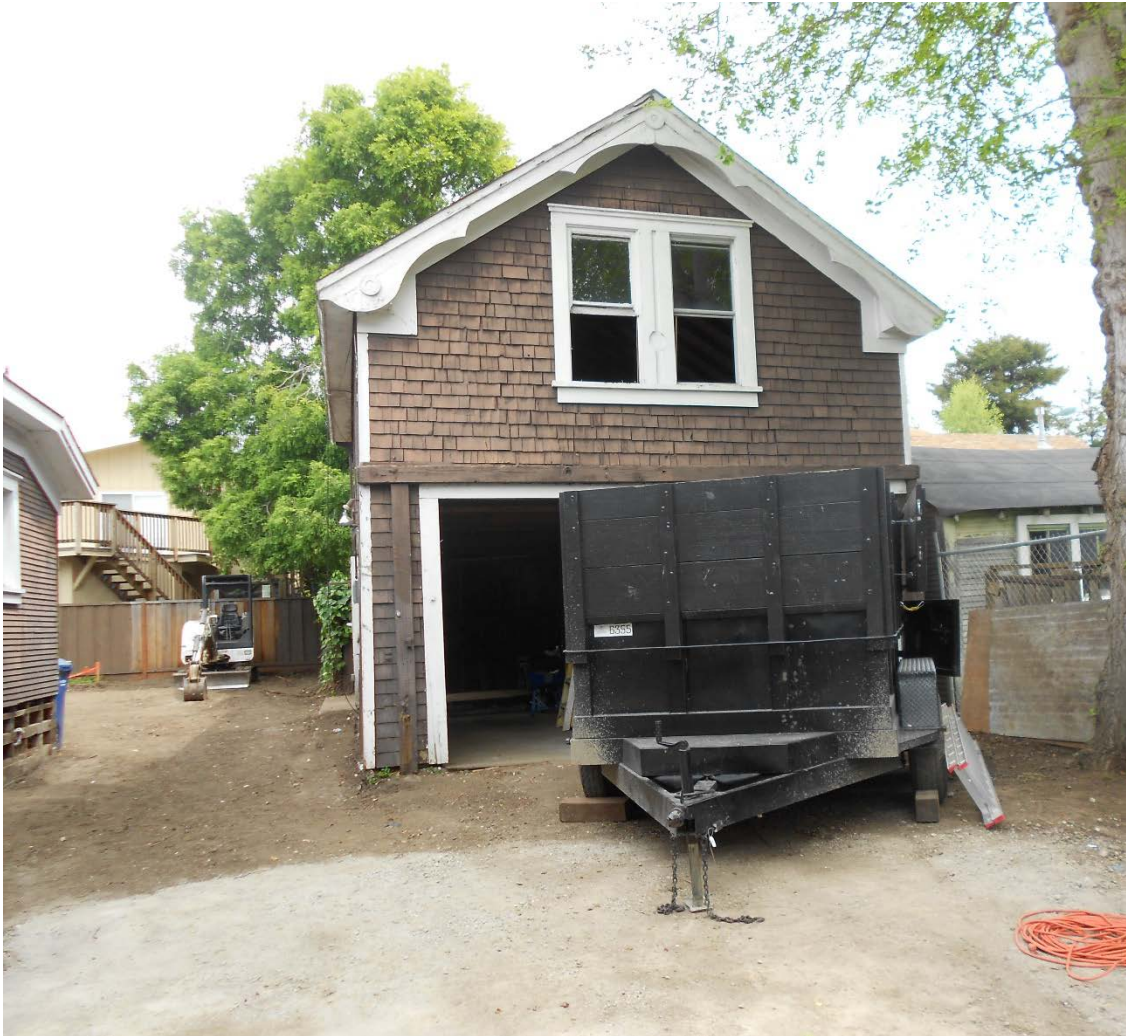
124 Central Avenue: Barn/garage c.1900 Note the sculptural cut of the bargeboard on the front and the enclosed eaves, detailing that is compatible with the house at 122 Central Avenue.
