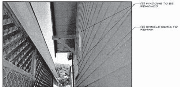
8 EXISTING SIDE ELEVATION - RESIDENCE SCALE NONE
