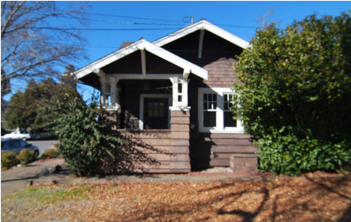
124 Central Avenue: South side of the double gable on the front porch.
