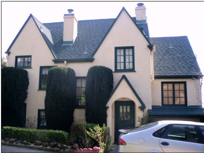
These buildings have several features that are characteristic of the Tudor style. Key features include multi-lite grouped casement windows, plaster, steep gable roofs and gable-roofed porticos.
